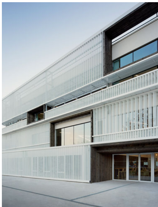
Fig. 12: Front detail view. © Takuji Shimmura.
