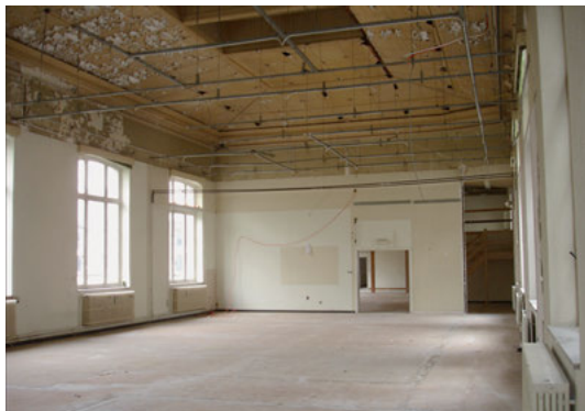
Fig. 4: Situation before the renovation was started. © UGent.
